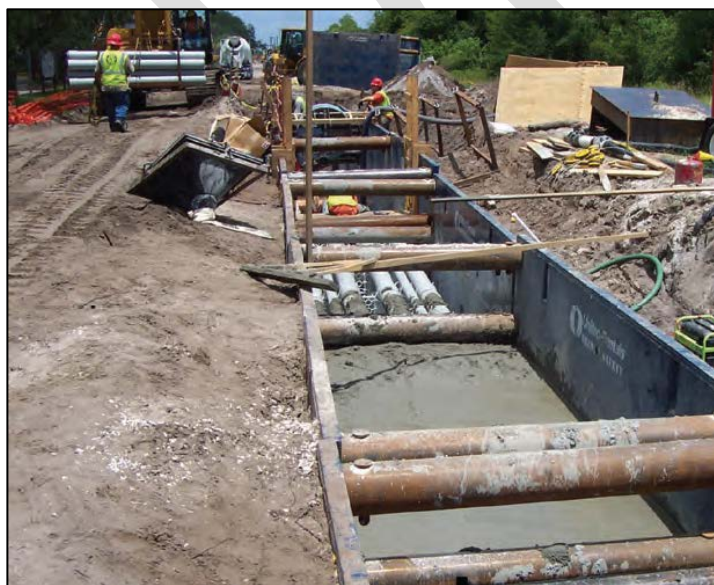
Figure 8. Underground power line construction (from APLIC 2012).
